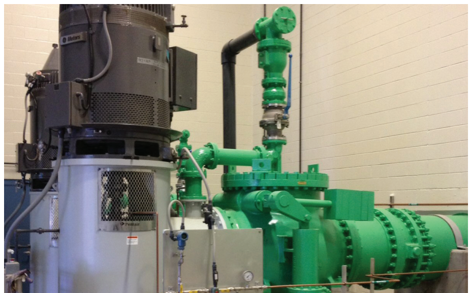
Columbia Canal Raw Water Pump Station, South Carolina — one 30" and one 24" Cushioned Swing Check Valve; one 6" and one 4" Figure 933-DK Air Valve.
