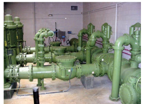
Raw Water Pump Station, Logan-Todd Regional Water, Tennessee — Three 16" Cushioned Swing Check Valves, Three 8" Figure 625-D Surge Relief Valves; Three 4" Figure 931-DT Air Valves.
