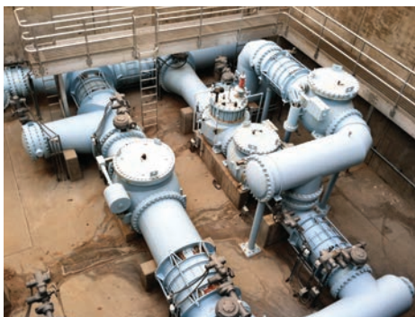
Happy Valley Reservoir, Arizona — Three 30" and one 42" Cushioned Swing Check Valves; One 30" Figure 3200-D Altitude Valve.
