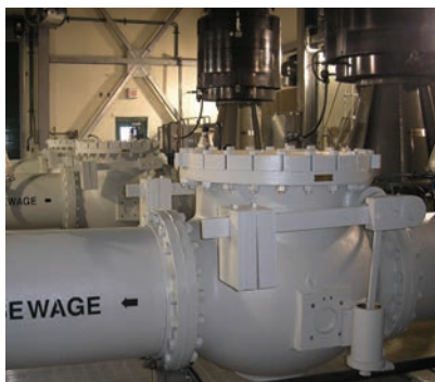
Influent Pump Station, Spring Branch WWTP, Alabama — Four 24" Cushioned Swing Check Valves.
