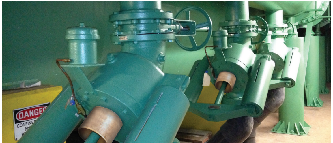
The new GA Surge Relief Valves installed at the Two Bridges wastewater management facility in Lincoln Park, New Jersey.
