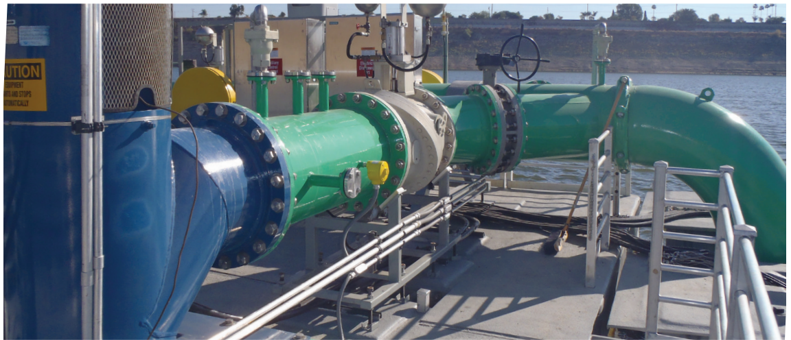
The GA Butterfly, Check, and Air Vacuum Valves installed on the floating pump station.
