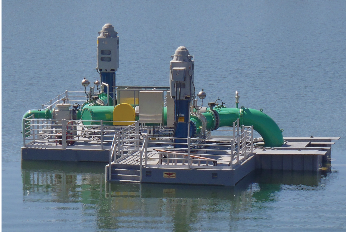
The floating pump station allows for the transfer of stored water from OCWD's Santiago Basins to other OCWD facilities.
