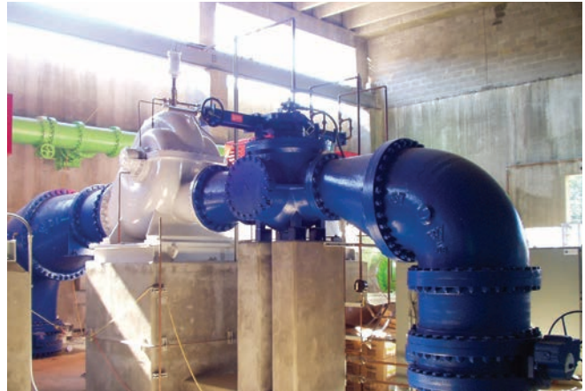
James T. Quarles Water Treatment Plant, Georgia, USA 2-16", 3-20", 2-36" GA Ball Valves with oil cylinder actuator
