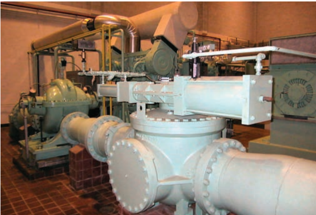
McLean Booster Pump Station, Saskatchewan, Canada 2-20" GA Ball Valves with air/oil cylinder actuator
