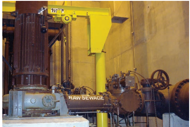
Meadowville Sewage Pump Station, Virginia, USA 3-12" GA Ball Valves with air/oil cylinder actuator
