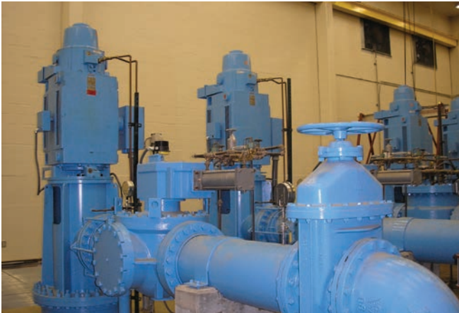
Etowah River Water Treatment Plant, Georgia, USA 6-16" GA Ball Valves with water cylinder actuator
